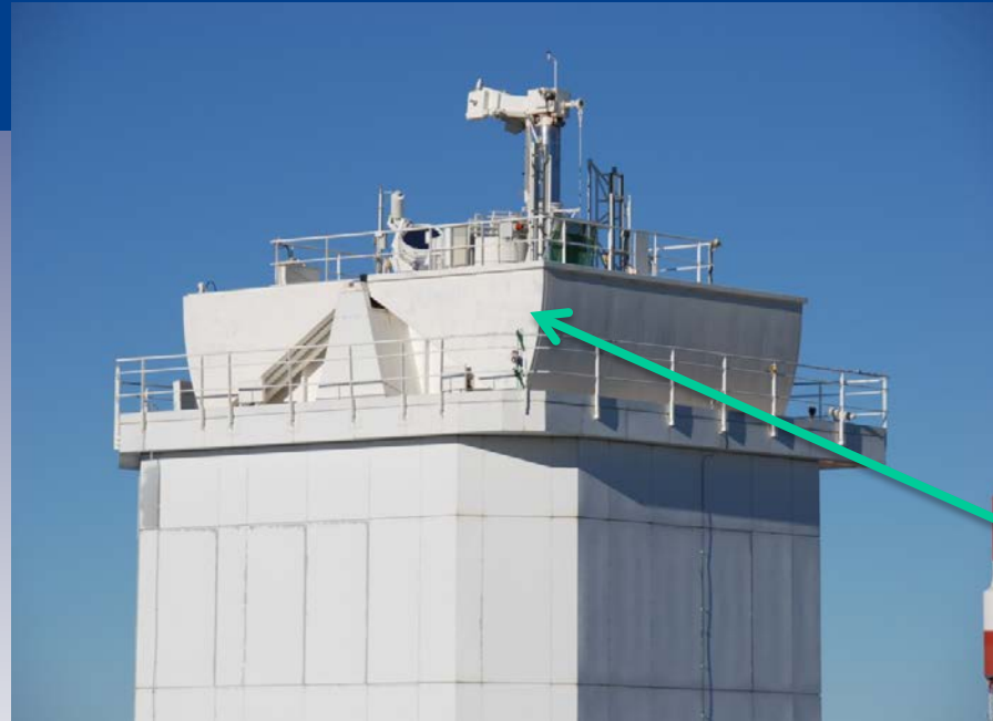
Transmitter at the VTT
