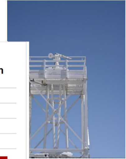
SHABAR AT OT ON TOP OF AN 8-METRE TOWER
