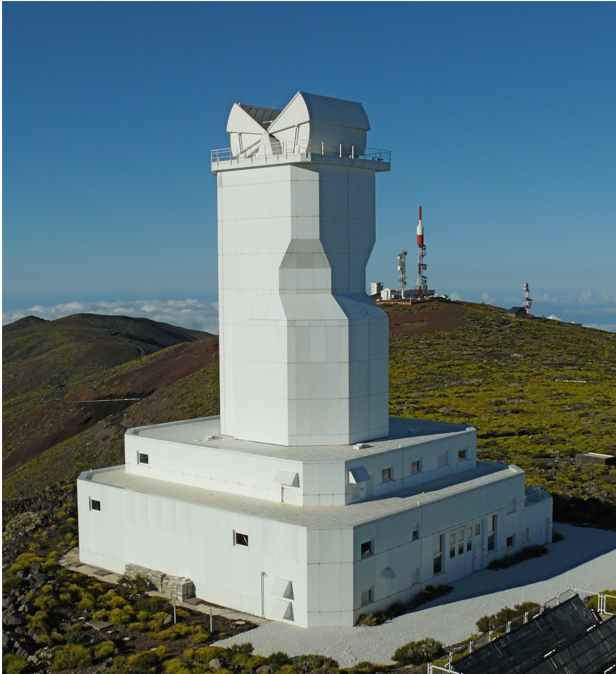
Fig. 1: The VTT seen from South-West, with partially opened dome (Foto W. Schmidt, 2007)
